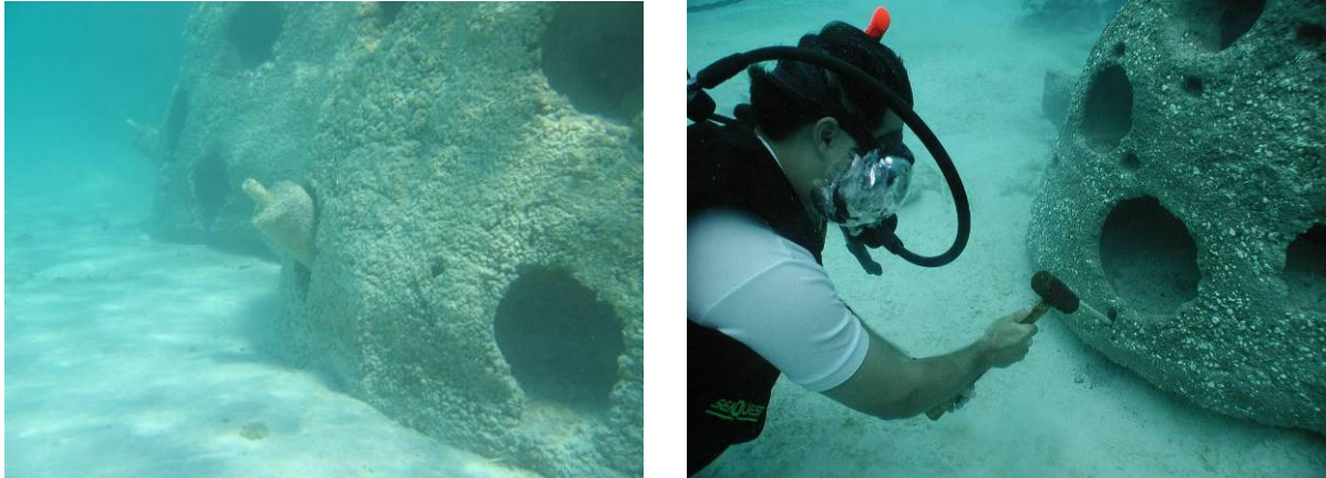
Figure 15. Pilings (left) and Rods (right) into Sea Bottom through Reef Ball Units
