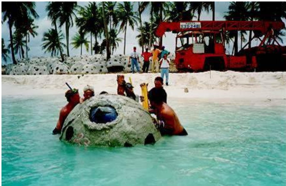
Figure 3. Deployment by Floating Reef Ball Units from Beach
